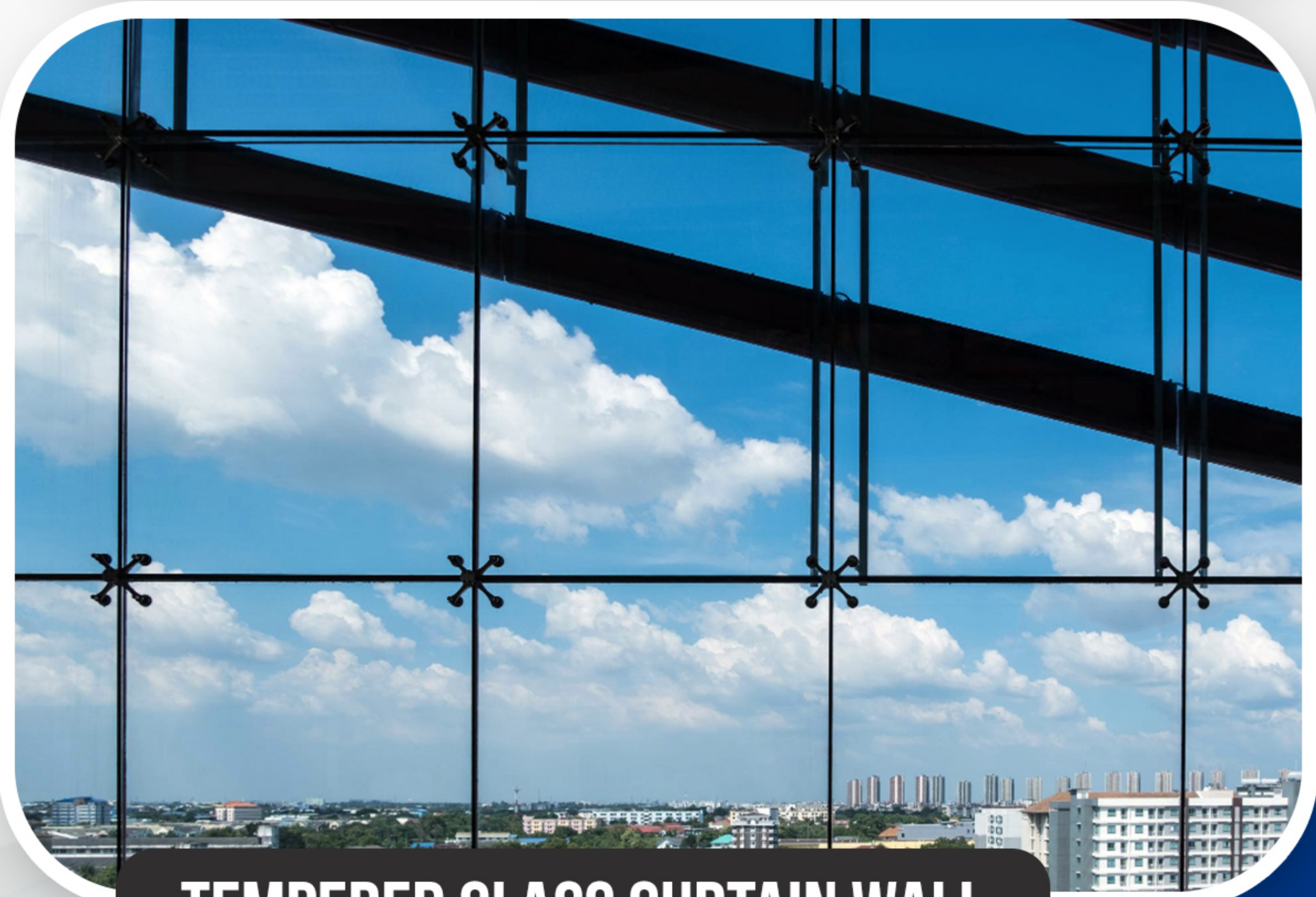
TEMPERED GLASS CURTAIN WALL
